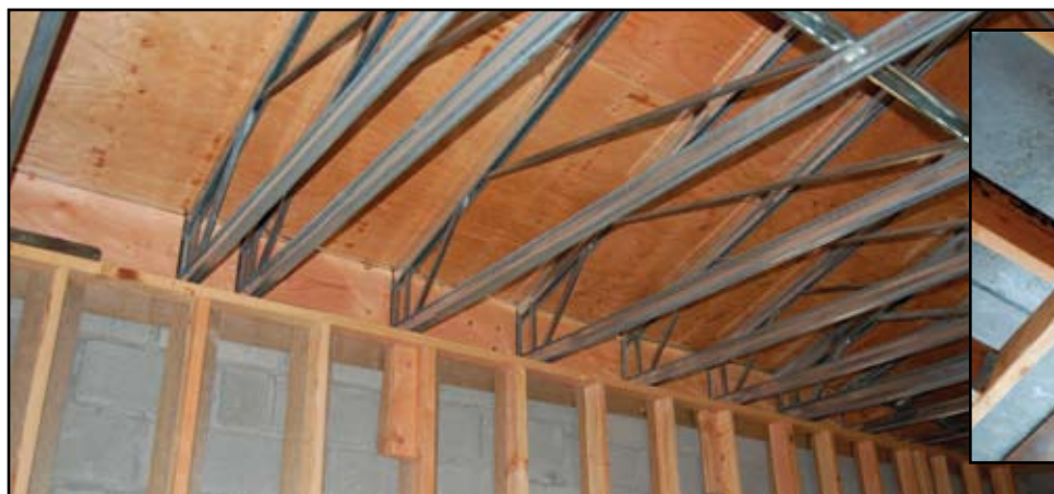
Roof Truss Diaphragm connection.
