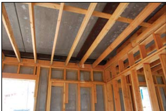
Spancrete with steel beam system.
