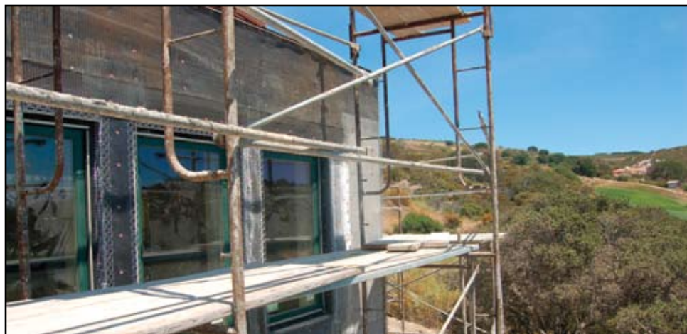
Exterior stucco application.
