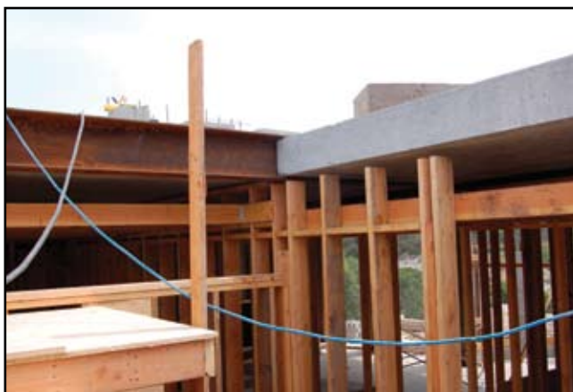
Second floor spancrete diaphragm.
