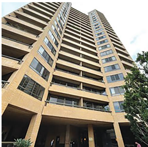
Figure 10 High rise building resting on 4 levels of subterranean parking.
