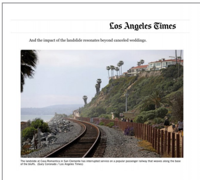
FIGURE 7: The main rail transportation link from San Diego to Los Angeles is blocked due to the landslide near Casa Romantica.
