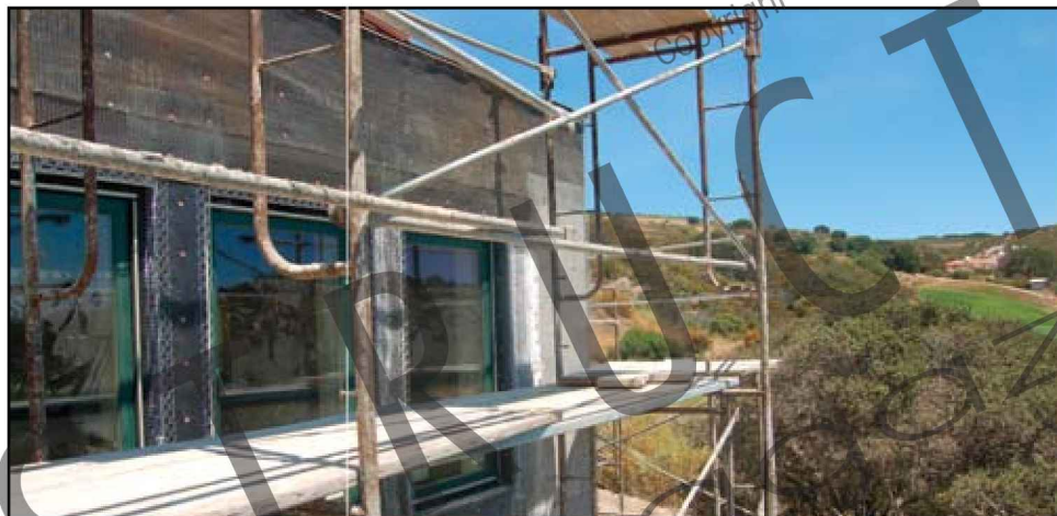
Exterior stucco application.
