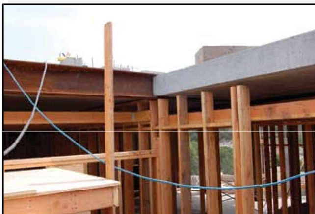
Second floor spancrete diaphragm.
