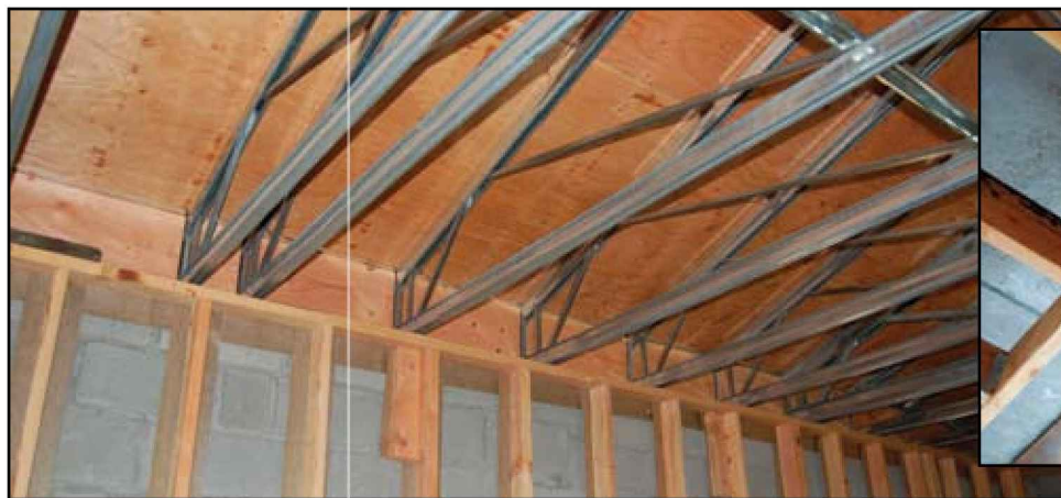
Roof Truss Diaphragm connection.
