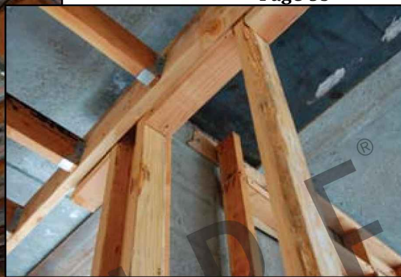
Interior non-structural wall connections.
